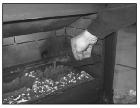
Figure 8.8 To remove the burner pan locators from the left and right sides of the burner, remove one screw from each side, lift locators up and out.
